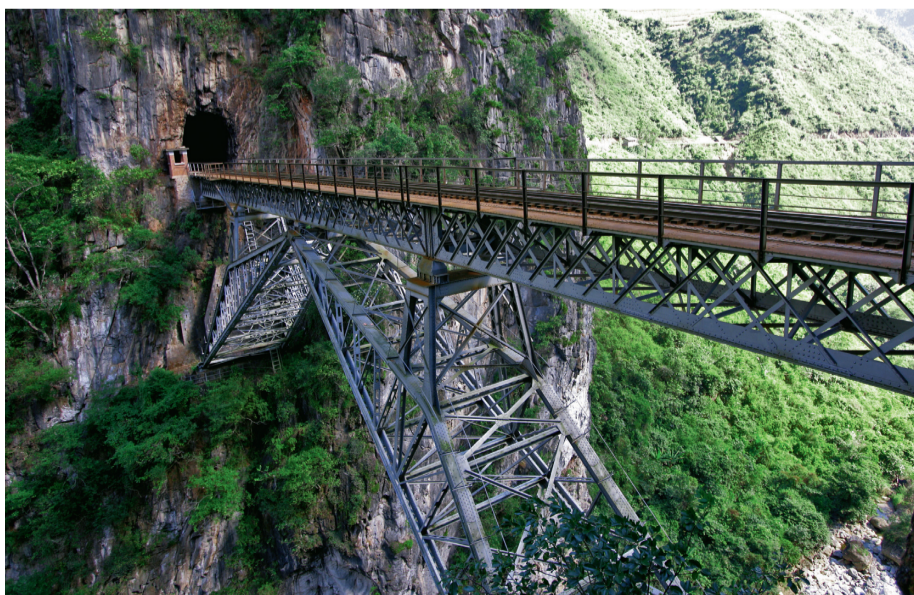
A view of the A-Shaped Bridge
