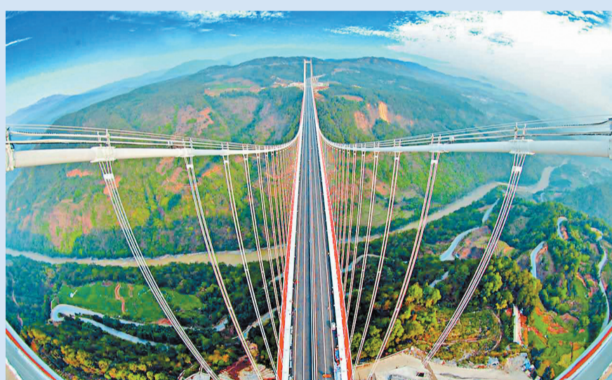
Asia's longest and highest bridge Longjiang Grand Bridge has finished closure in advance and passed load test on April 5. The 8,100-foot-long suspension bridge over Longjiang River, southwestern China's Yunnan province, will open to traffic on May 1, 2016. The new bridge, connecting the cities of Baoshan and Tengchong, and going straight to Myanmar.
