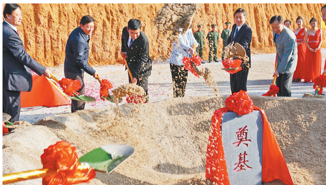
The foundation-stone laying ceremony of the Lancang-Mekong International Vocational Institute on December 17.
