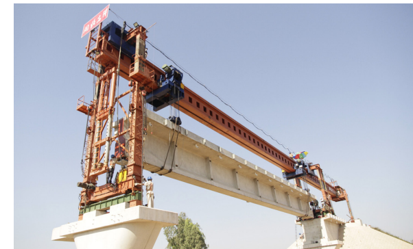
A bridge-building crane works on the China-Laos Railway.
