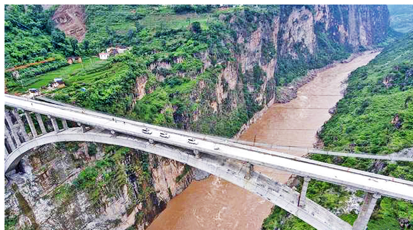
The newly-built Yingge Bridge in Qiaojia County, northeast Yunnan (Photo by Xinhua)
