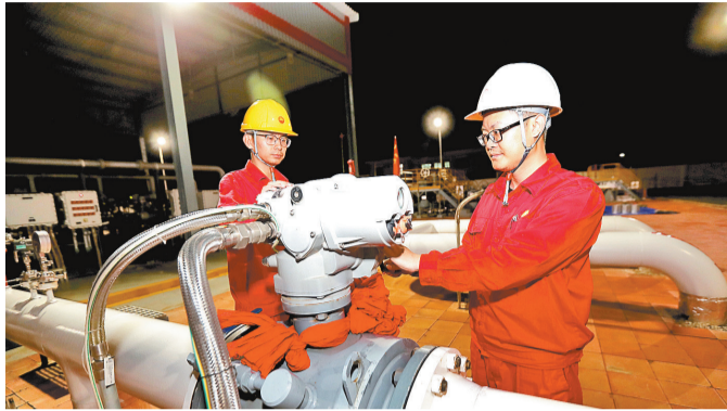
Workers open the valve of the Kunming branch line. Xinhua photo
