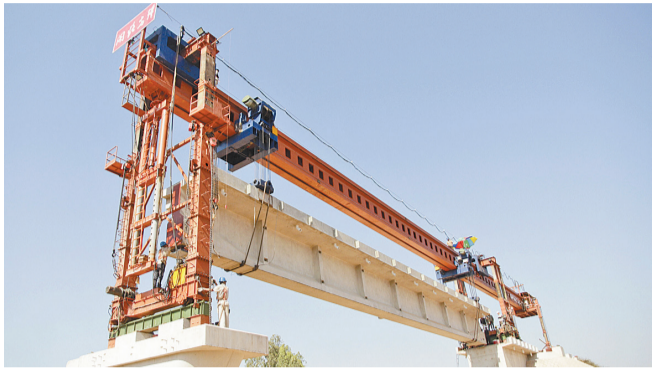
A bridge-building crane works on the China-Laos Railway. (Xinhua)
