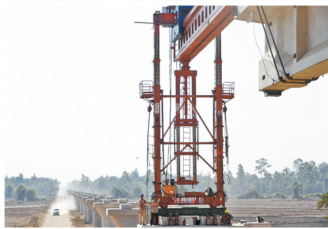
Construction site of China-Laos Railway.
