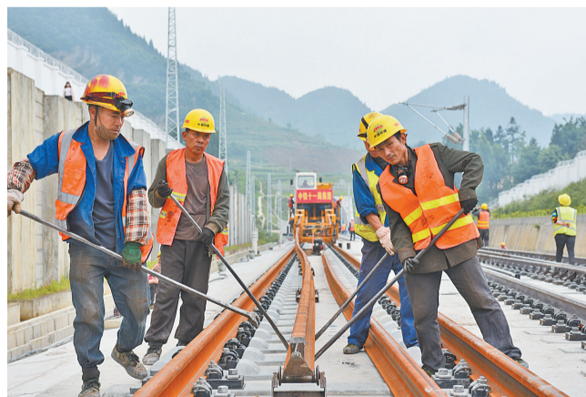
Workers are laying tracks for the railway.
